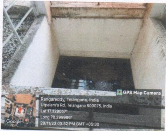
WASTE WATER WILL BE SWEEP IN TO THE GROUND / VEGETATION THROUGH THE GRAVEL
