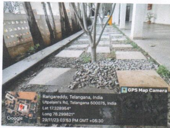
WASTE WATER WILL BE SWEEP IN TO THE GROUND / VEGETATION THROUGH THE GRAVEL
