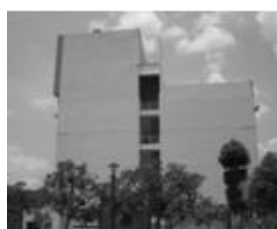
Building façade facing to the east
