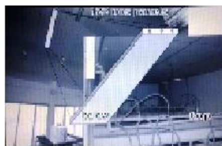
Chilled metal ceiling (CMC)
