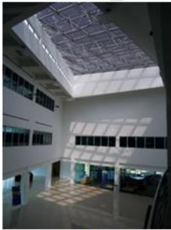
Atrium with glass semi-transparent PV modules (11.64kWp)
