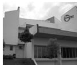
Building façade facing to the west
