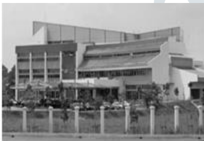
Building façade facing to the north
