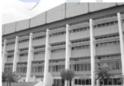
Building façade facing to the south
