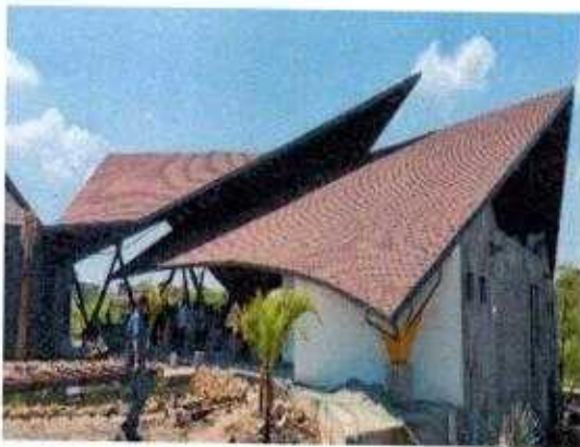
Roofing system of activity centre
