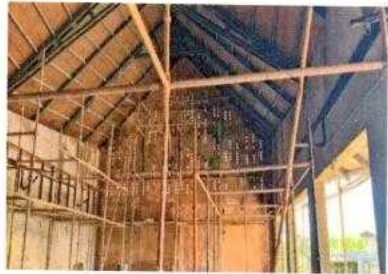
Glass bottles used in between the walls
